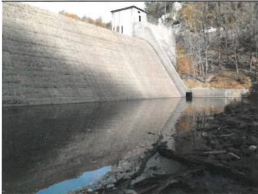
North wing wall of the Roxbury Dam
